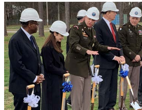
Honorable Ronald Moultrie, Under Secretary for Intelligence and Security (left) joins others in breaking ground on an expansion to DIA's Missile and Space Intelligence Center in Huntsville AL.
